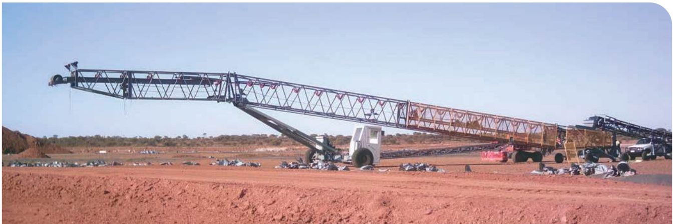
Figure 7: Heap leach conveyor stacker example
