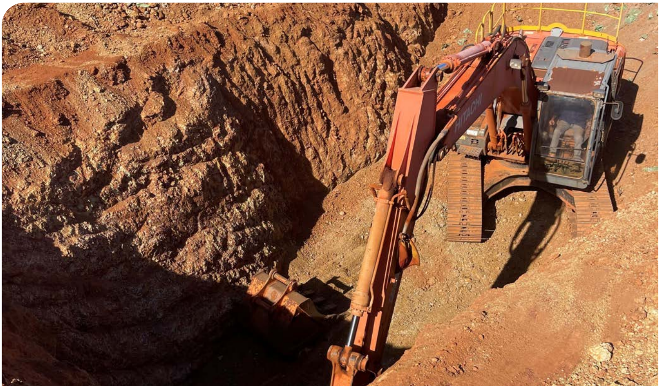
Figure 5: NiWest Project site activity
